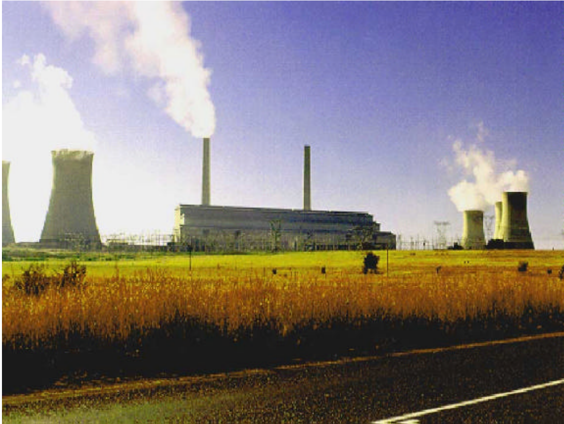
Figure 1: Hendrina Power Station after phase two. One chimney ESP's and one chimney FFP's
