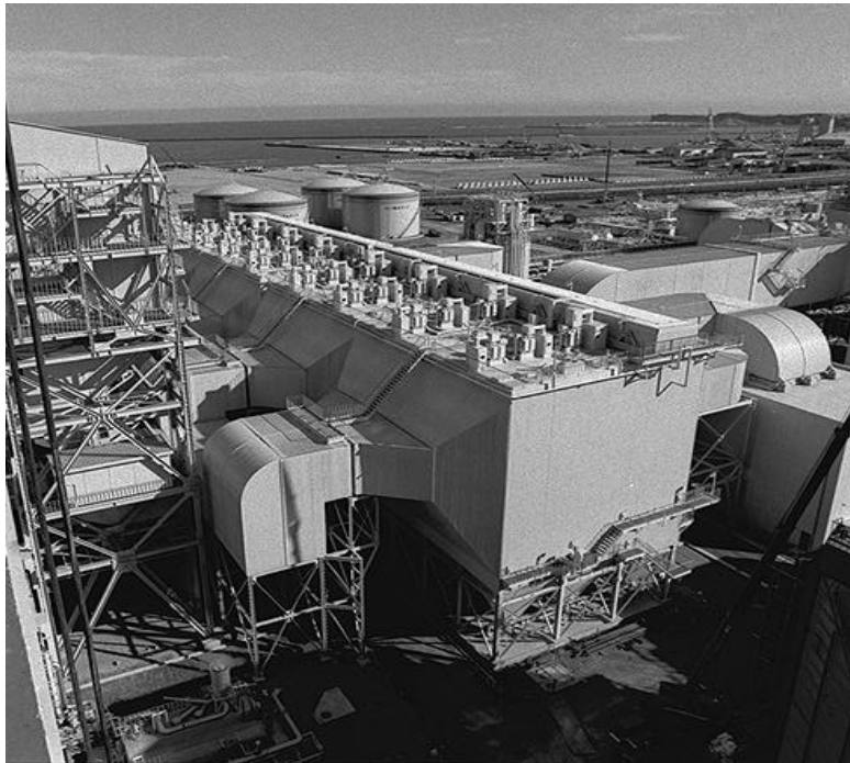
Fig. 1 Application of MEEP for 1000MW Coal Fired Utility Boiler
