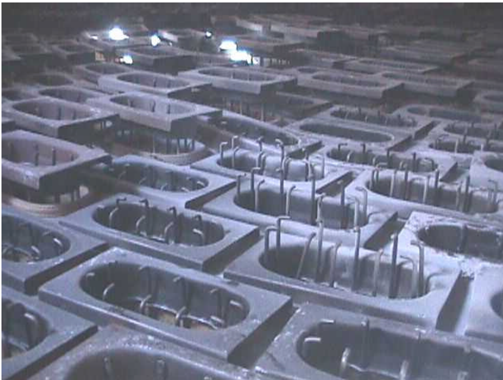
Figure 1: In the above photo the two types of cages can be seen. The highest telescopic cage (MK1) in this photo is 42mm above the tube plate and the highest normal cage is 97mm, although the bag shrinkage is virtually the same.
