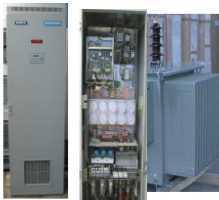
Figure 4: IGBT HV power supply 200 kVA
