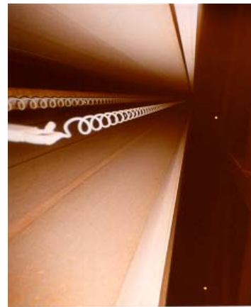
Figure 4. Emitting and collecting electrodes of the new ESP
