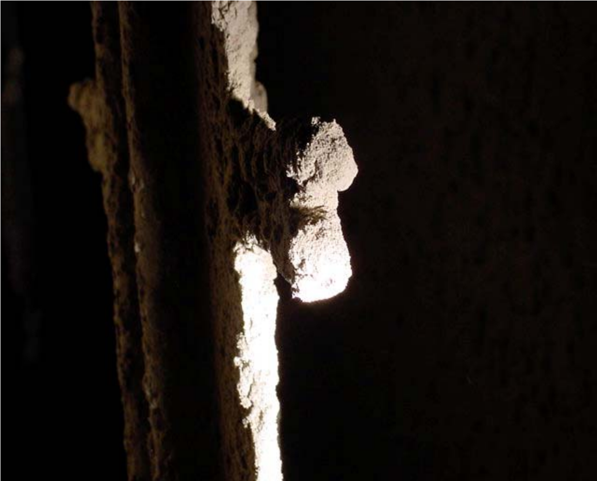
Figure 1 Fouled discharge electrode resulting from an economiser tube leak.
